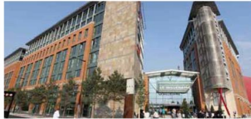
Partitions and doors - «Le Millénaire» shopping centre Aubervilliers, France
